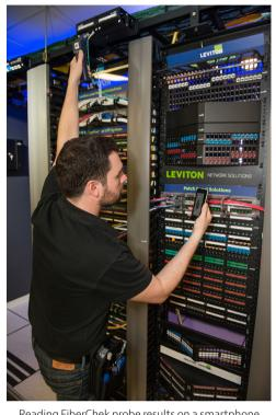
Reading FiberChek probe results on a smartphone
